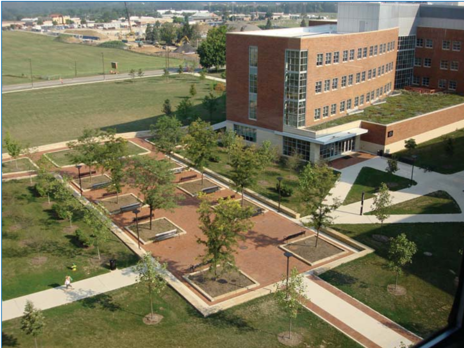
Figure 2. Forest Resources Building, Penn State University campus.
